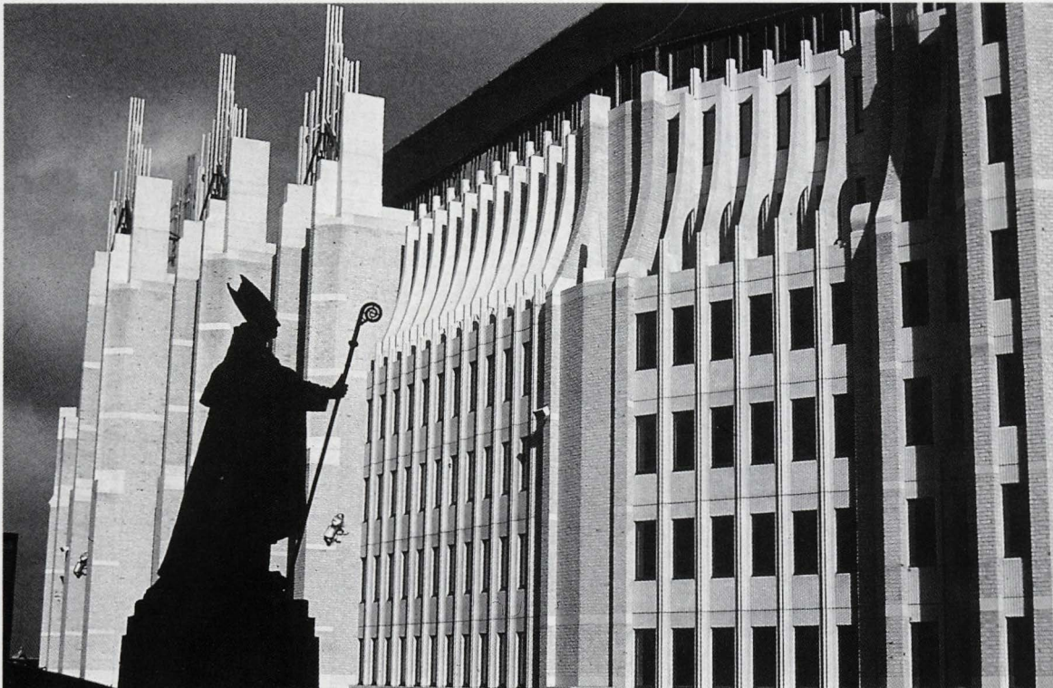
Markiescomplex, Brussel Architect André Jacqmain / Atelier de Genval 1985-1990
